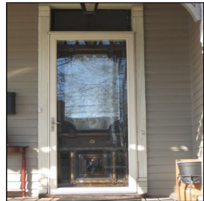
Installing full-view storm doors for energy conservation is appropriate (410 S. First Street).
