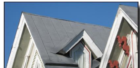
Preserve and maintain original metal roofs (422 S. First Street).
