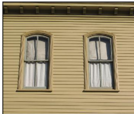
Original two-over-two wood sash, arched windows.
