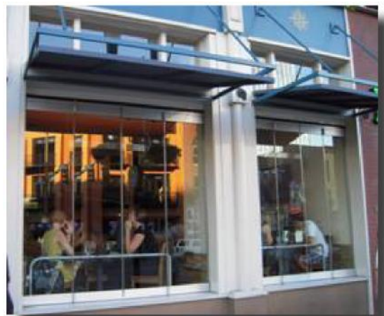
Side-hinged retractable windows on infill building.
