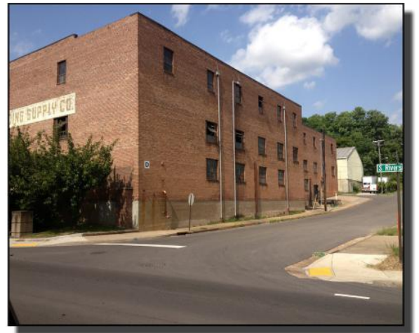
Example of multi-story commercial building.
