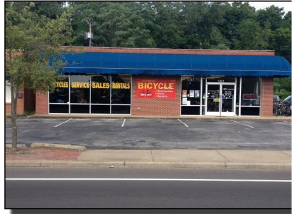
One-story brick commercial building on Riverside.
