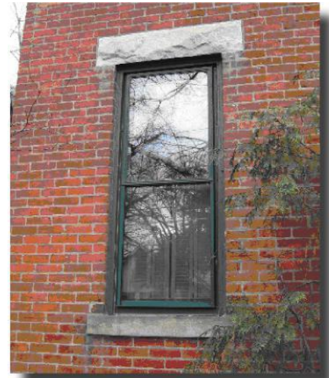
Storm windows should be full view design or match the meeting rail of the window.
